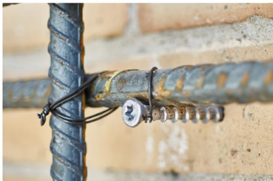
FIGURE 7 – PYTHON MT MANUFACTURER'S PUBLISHED INSTALLATION INSTRUCTIONS FOR NEW CONCRETE/SHOTCRETE TO STARTER-BAR (MPII)
