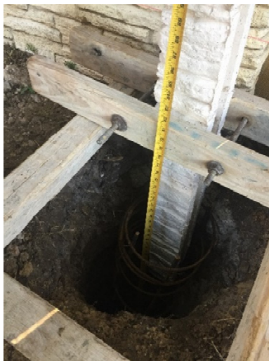
Figure 6: Post to Foundation
