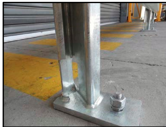
FIGURE 2—TYPICAL BASEPLATE ATTACHMENT
