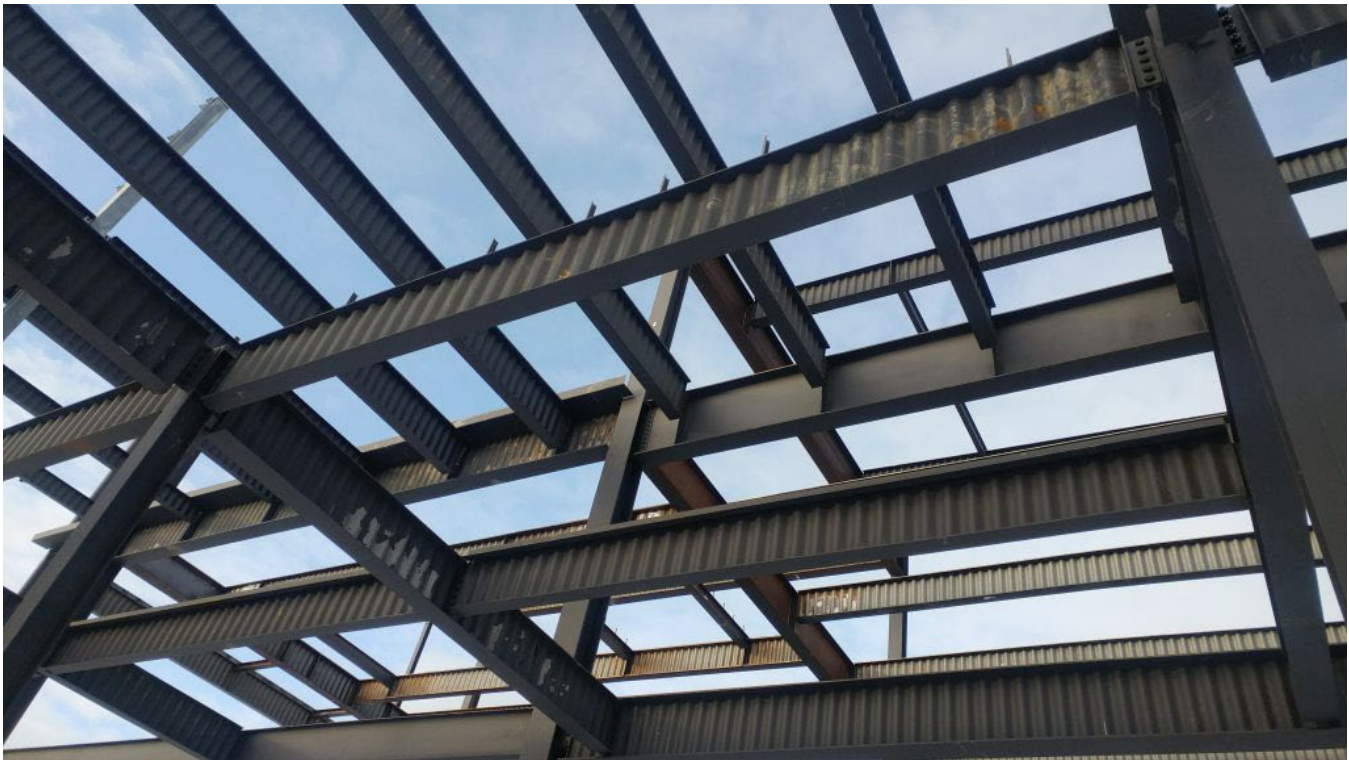
FIGURE 1—SIN BEAM FRAMING
