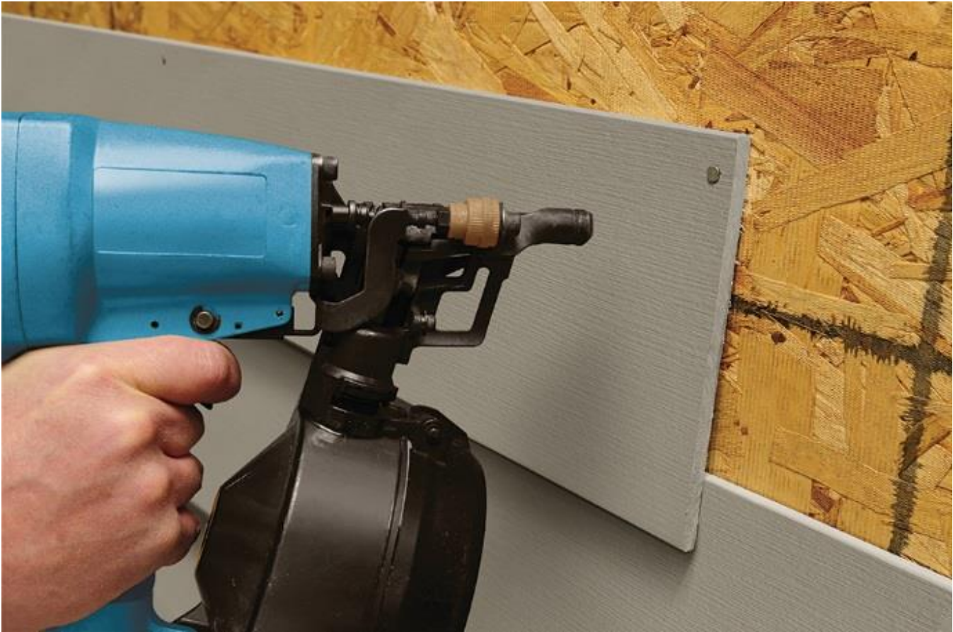
FIGURE 2—EOTEK SIDING INSTALLATION
