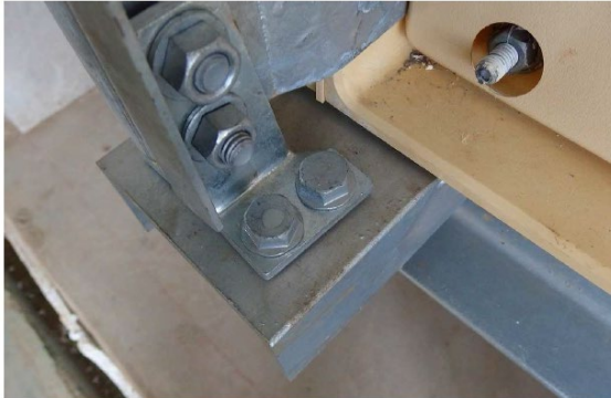
5C LOWER BLOCK ANGLE CONNECTION (2M TANK)
