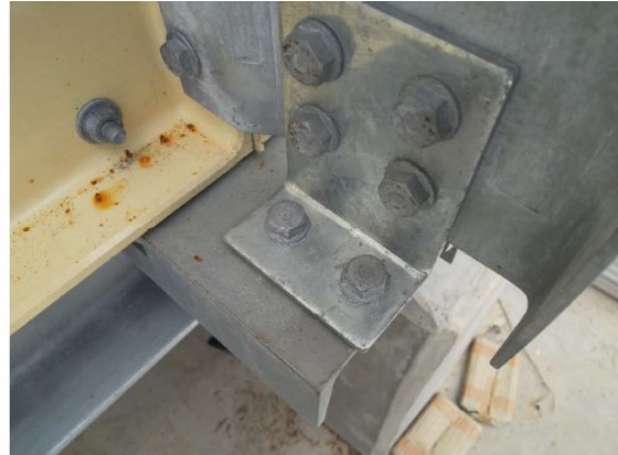
5B LOWER BLOCK ANGLE CONNECTION (3M TANK)
