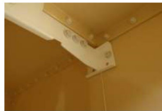
2B INTERIOR ROOF MEMBER
