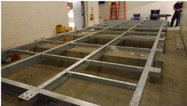
6A STEEL FOOTING ASSEMBLY
