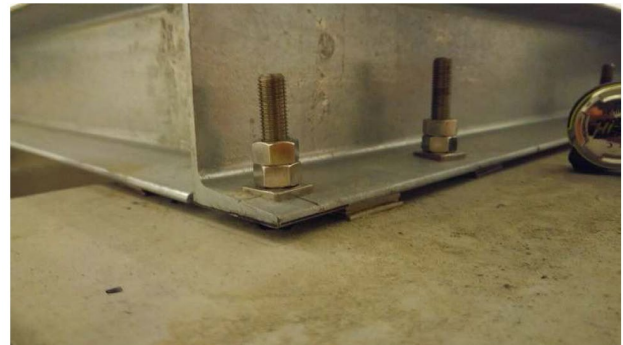
5D STEEL FOOTING ANCHORAGE
