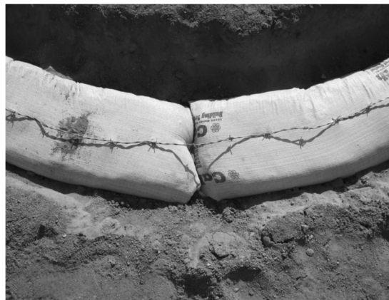
FIGURE 1—CALEARTH SUPERADOBE EARTHBag WITH BARBED WIRE PLACED AT STACK INTERFACE OF COURSES
