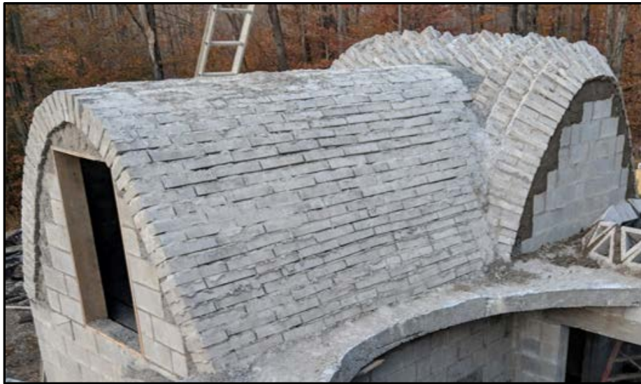
FIGURE 4 – SMOOTH ARCH (LEFT) ABUTTING A CORRUGATED ARCH (RIGHT)
