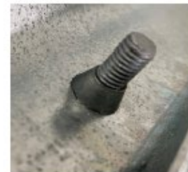
After break away nut is installed
