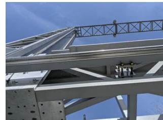
3D printed concrete wall construction (photo courtesy of Black Buffalo 3D)
