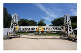
Black Buffalo 3D Concrete walls are structural walls - printed with NEXCON 3D automated construction technology and Planitop 3D - used as bearing walls, non-load bearing walls, and shear walls in multi-story structures. Black Buffalo 3D Concrete walls are an alternative to concrete walls as described in ACI Code 318, and as permitted by Section 104.11 of the IBC. More information can be obtained from ESR-4623.
