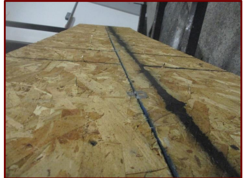
Fire-Retardant Penetrant – Nail Penetration through the Surface, No Delamination, NOT a coating!
