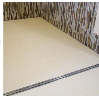
His "better way" is a one-way slope that is based, he says, on simple math and physics. It can shave hours off of installation time and is much easier all the way around, he said. "In a recent building project, we saved the contractor \$150,000 on time and labor costs."
